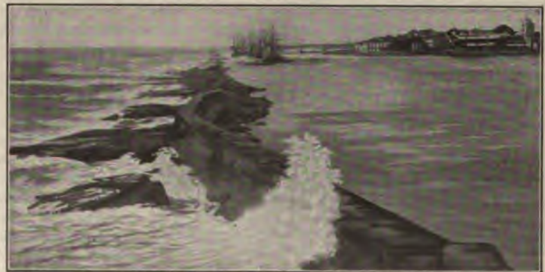
The harbor of Pernambuco, showing the natural reef which has been extended by a sea wall so as to give the city a harbor.
